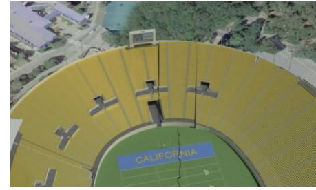
California Memorial Stadium straddles the active Hayward Fault in Berkeley, California.
